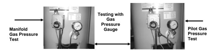
Gas pressure checks are done with flowing gas.
